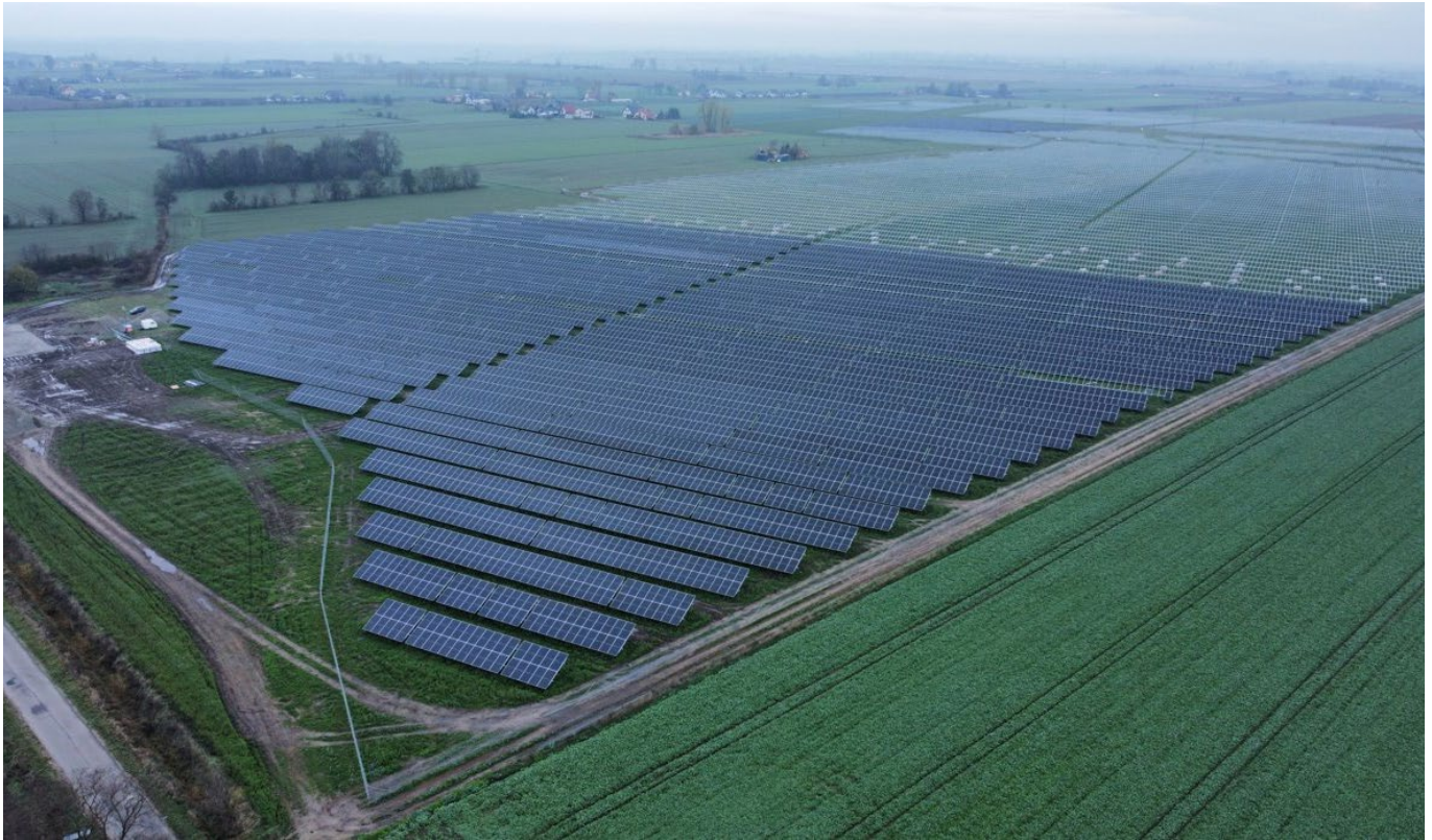
Construction status of the Kleczew Solar & Wind project – November 2022
