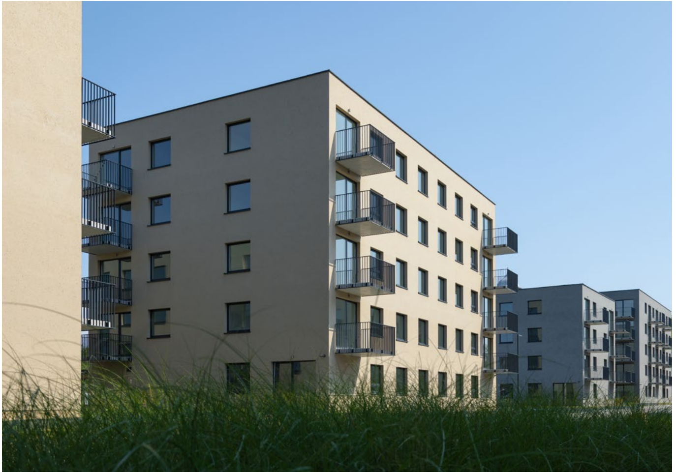
The Housing Development Fund, Katowice, ul. Korczaka, 524 apartments
